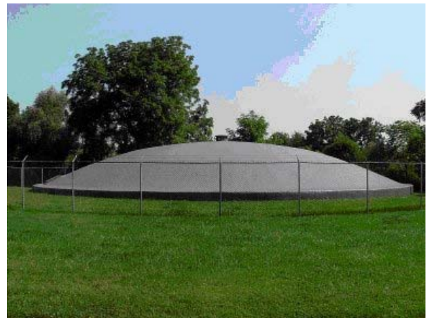
Water tank where the SmartBall was inserted into the Schantz Spring Pipeline for the City of Allentown
